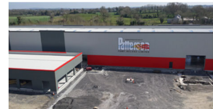
Patterson Pump Ireland
