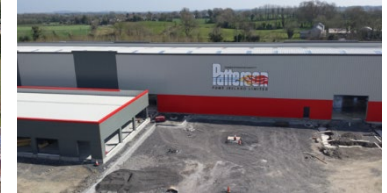
Patterson Pump Ireland
